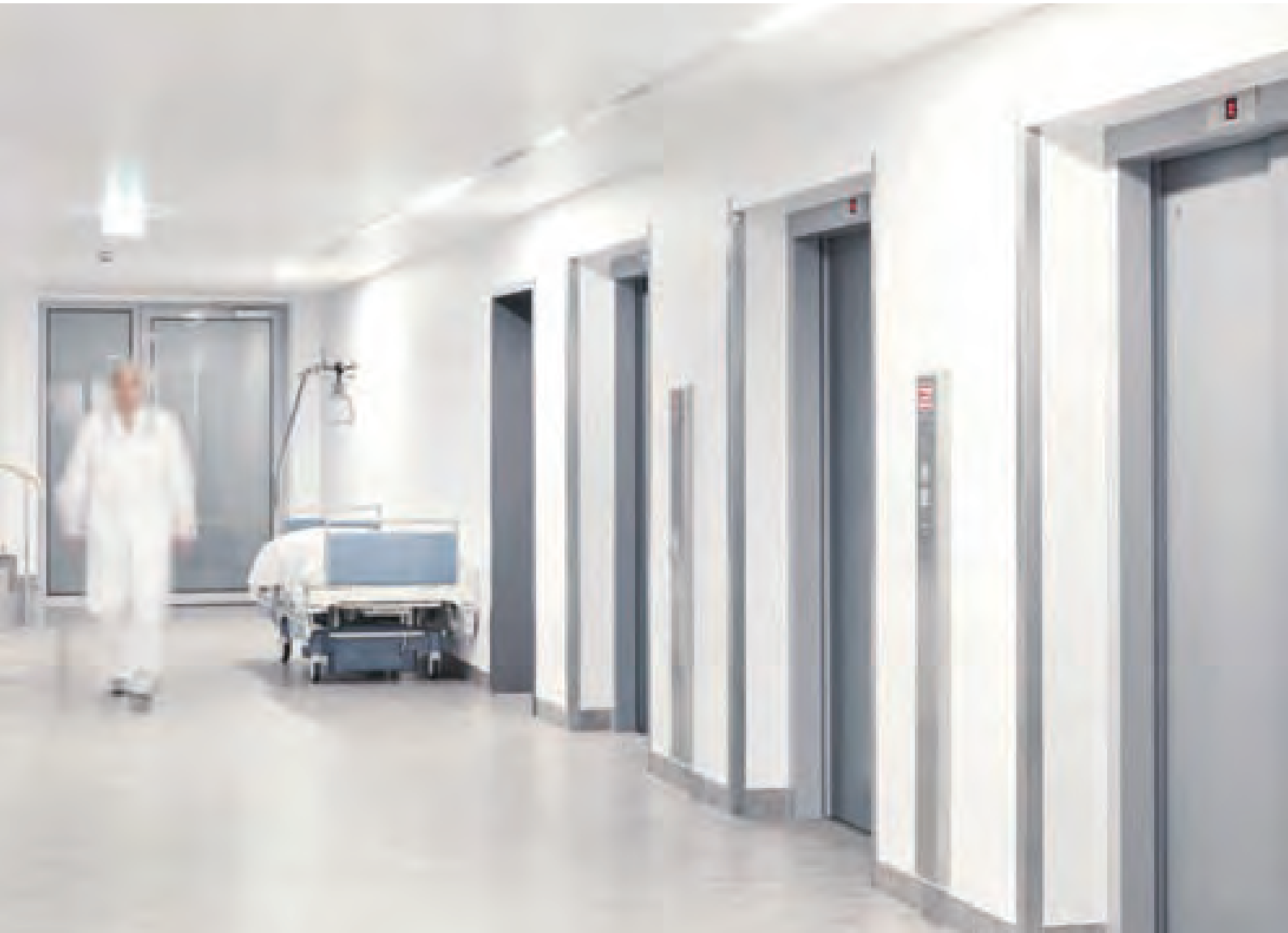
A TYPICAL COMMERCIAL ELEVATOR USED IN HOSPITALS
