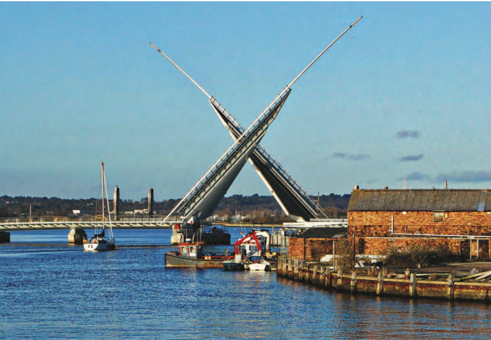
DOUBLE LEAVED BASCULE BRIDGE
